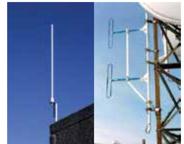
Omnidirectional (left) and offset dipoles (right) serve as data receptors for the dispatch control center
